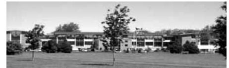
Kings Regional Rehabilitation Centre
